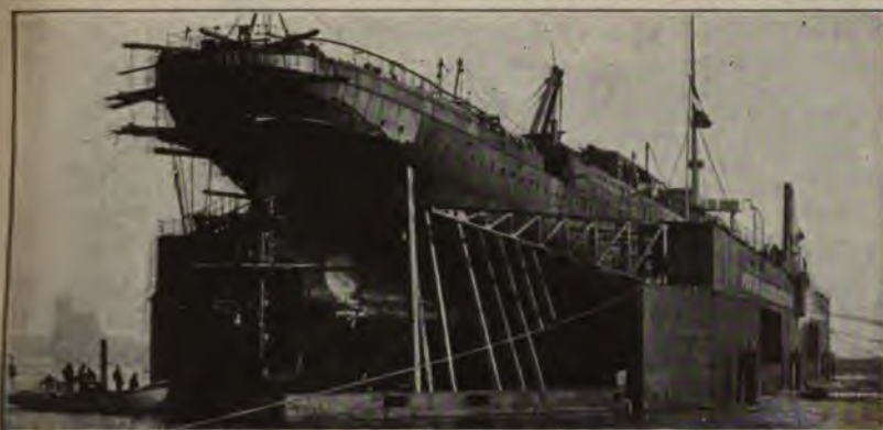
An ocean steamship in dry dock at the Vulcan yards, Stettin.
